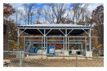
The foundation slab and structural steel have been erected and installed for the new Grounds Garage. The concrete pad and bollards have been poured and installed in Parking Lot 3 for the new aboveground fueling system. The anticipated completion for this project is on schedule for February 2024. This project is funded through the College's Chapter 12 appropriation.
