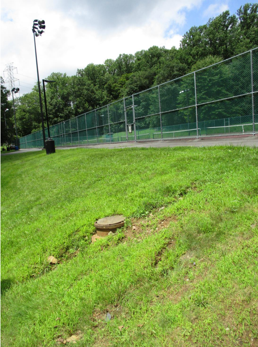
Sewer/Water system manhole
