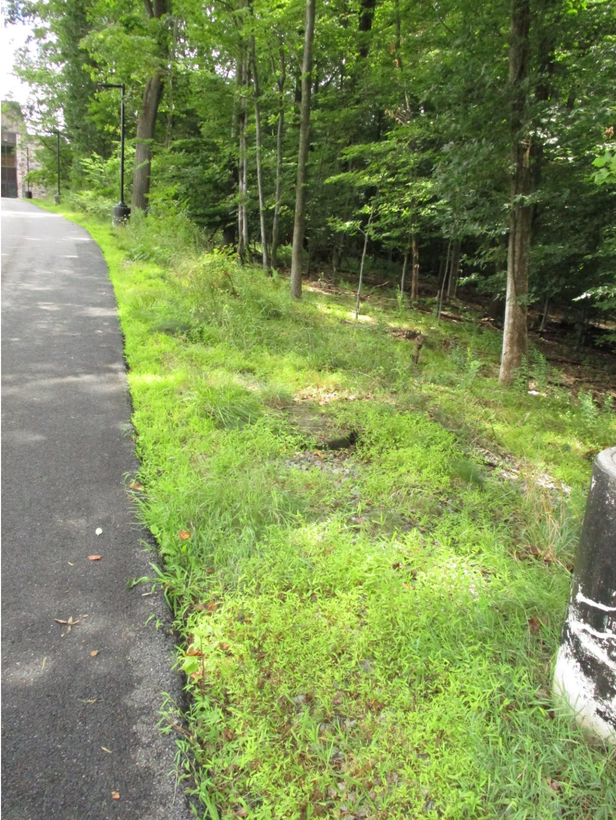
Manhole right of driveway to HPE from Pavilion
