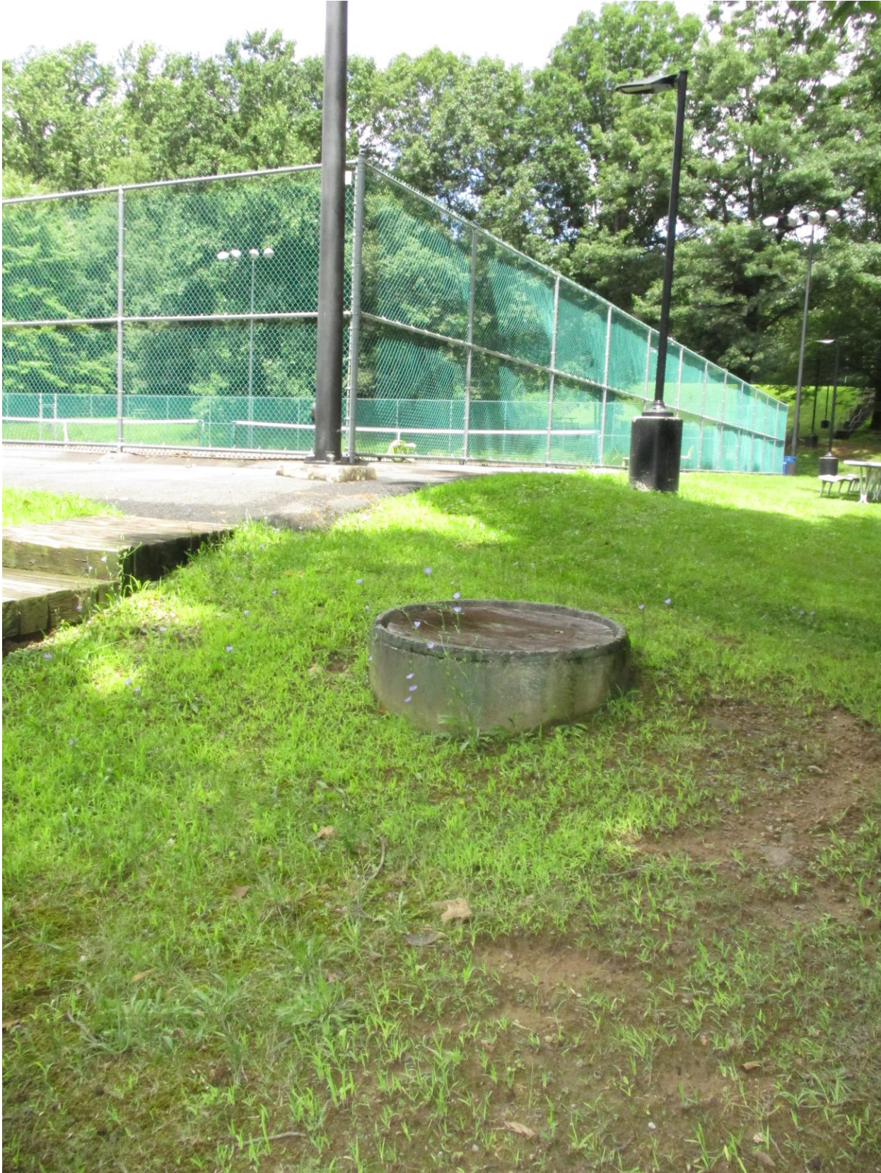
Sewer/Water system manhole
